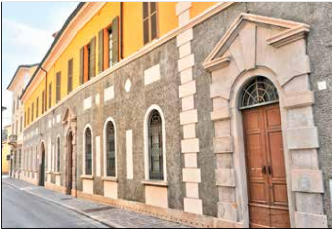
Figure 8. Entrance to The A&C Azzini Velocipedes and Antique Bicycles Museum in the Vertua-Robbiani Palace in Soresina.
