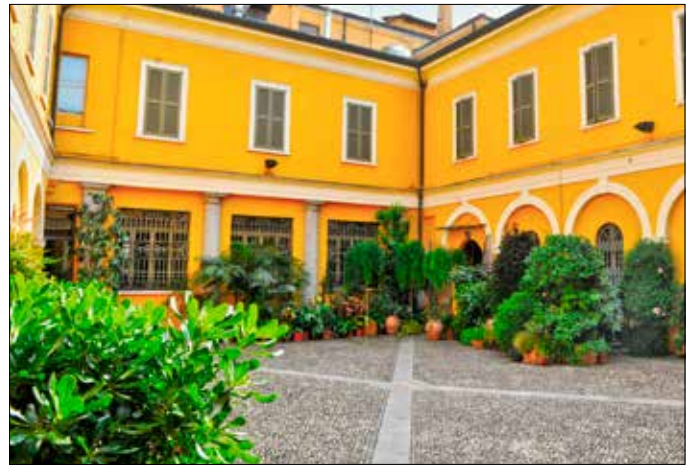
Figure 9. Internal courtyard to the palace.
