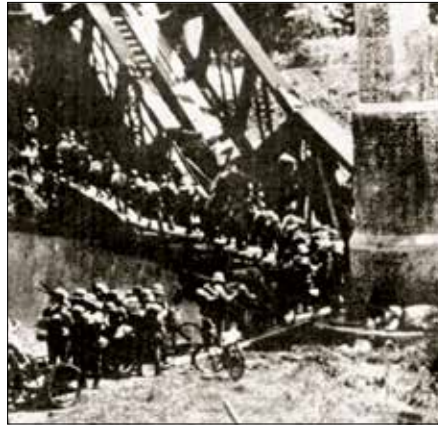
Figure 7. Cyclists among troops crossing an improvised walkway alongside a railway bridge destroyed by the British, possibly the Guillemard bridge near Machang, Kelantan. (USAMHI)
