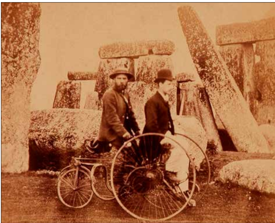
Figure 8. NO CHAIN ... NO ROOF ... NO WORRIES Duplex Excelsior D. D. (Double Drive) tandem tricycle made in England. Photograph circa 1883. Genre in the market for but a short time (circa 1881–1885). Open front, rear steering adult tricycle. Cog driven (chainless). Independent double driving. Built by Bayliss, Thomas & Co. of Coventry. Considered the first successful tandem tricycle. (Tricyclists' Indispensable Annual, 1883, Sturmev, pgs. 177–178). Captivating image taken at Stonehenge. For years one could wander throughout the site. Today it restricted to entry. Unknown English photographer. Albumen Cabinet card.
