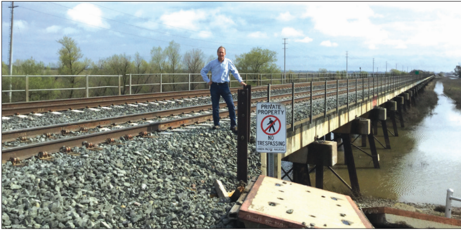
Figure 3. The railway trestle traversed by Thomas Stevens. (Photo by the Author).
