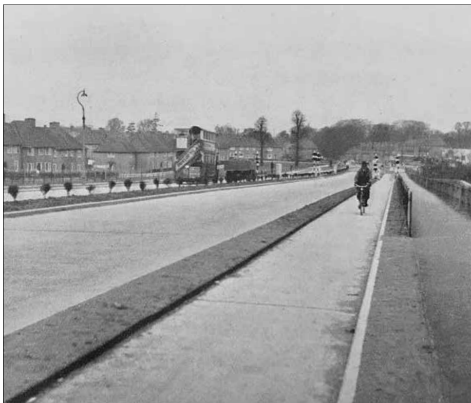
Figure 3. Shown here is an example of a concrete cycle path in the London area that has been finished with a solid, smooth surface for comfortable cycling.
