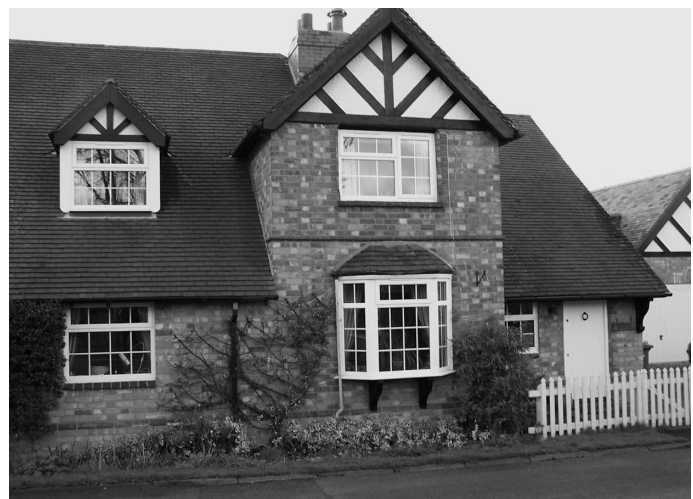
Right: Fig. Lawrence 5. Ladbroke Tollhouse as it appears today (2007).
